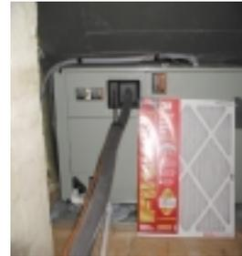
High efficiency furnace filter
